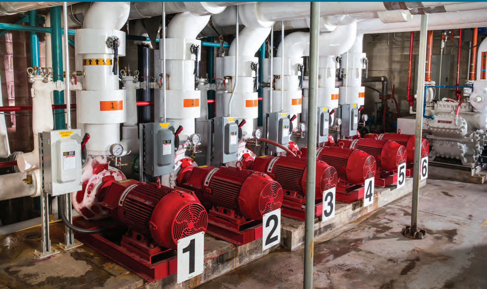
Max efficiency and control - glycol pumps with variable frequency drives each feed a specific rink
